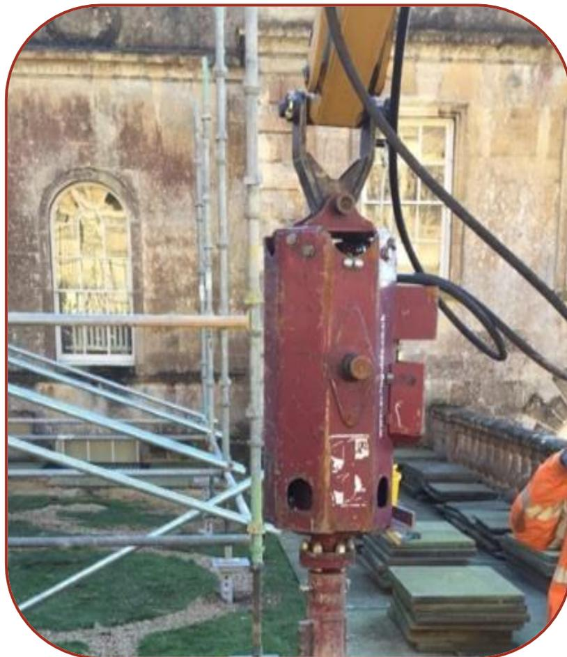
4. De-pressurise hydraulic systems using the manufacturers approved techniques before connecting the Powerhead.
